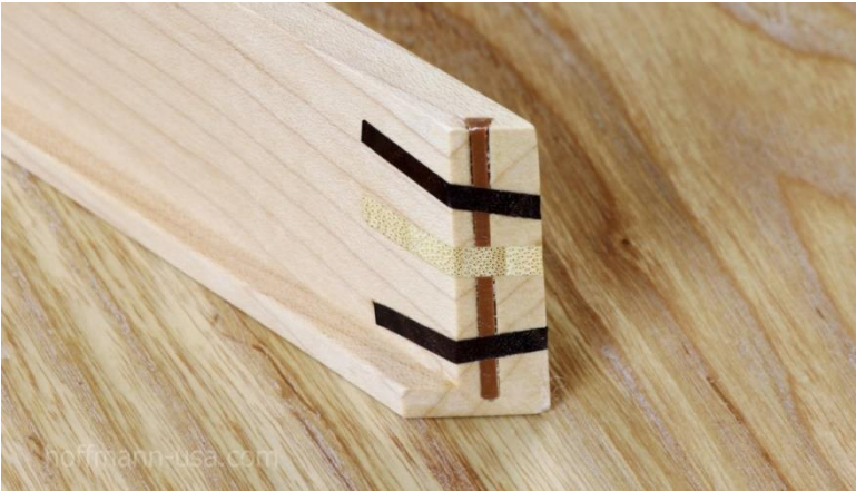
Cross-section of maple picture frame moulding with W-1 plastic Key and walnut and bamboo splines
